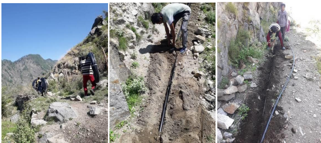
Figure 31. Carriage and laying of HDPE pipes.
