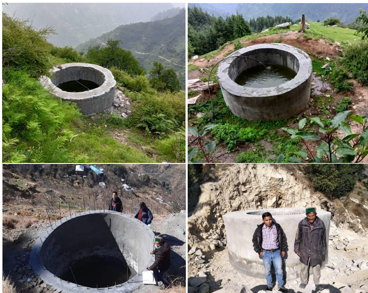
Figure 32. Water storage tanks constructed under the Project.
